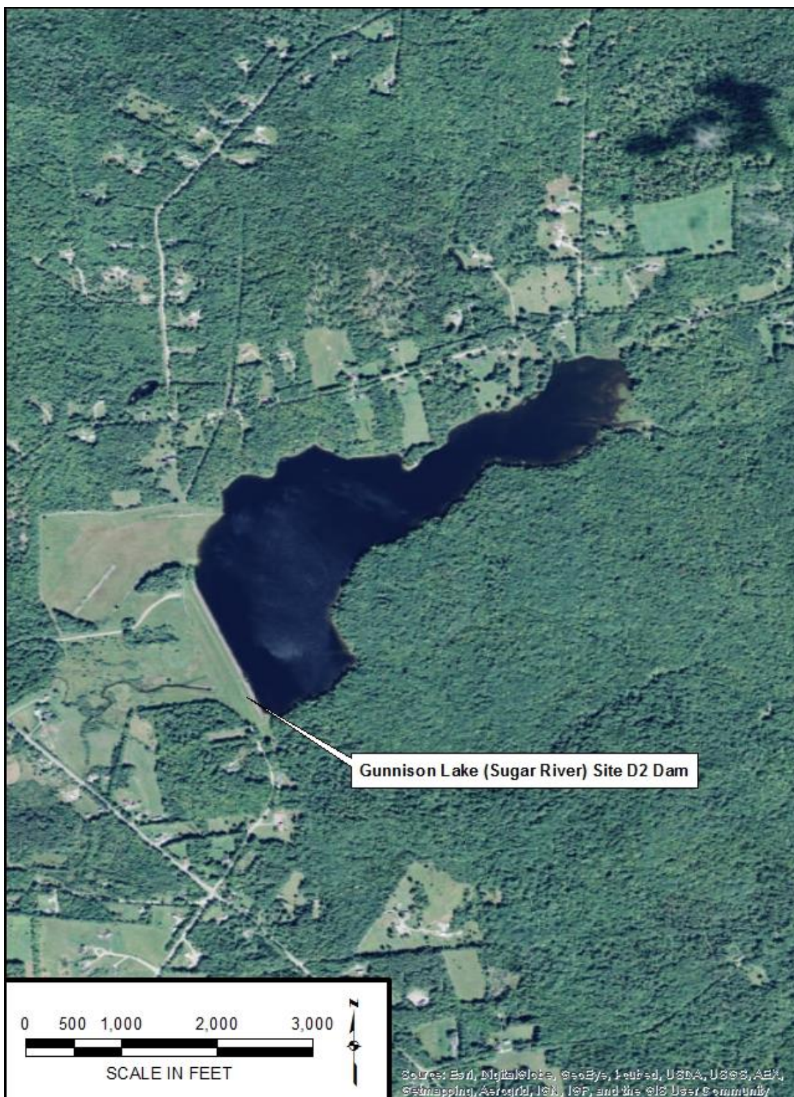
Figure 1. Aerial photograph of Sugar River Site D-2 Dam
